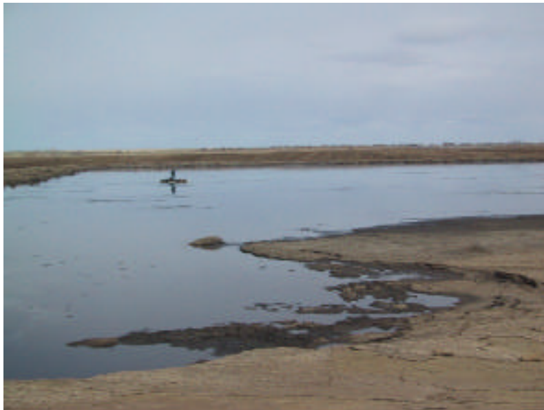
Partially Empty Primary Holding Pond Showing Sediment
