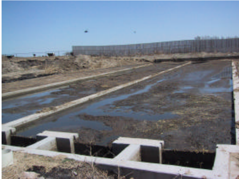
Floating Solids on Top of Gravity Separator
