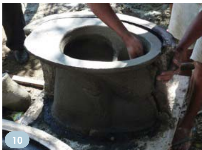
Pic 9/10: Construction of Urine Diversion Concrete Bowls (by WAND Foundation, Libertad)
