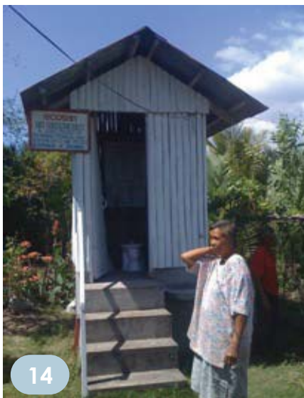
Pic 14: Urine Diversion Dehydration Toilet (Bayawan)
