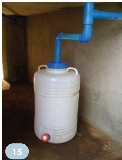
Pic 14: Urine Diversion Dehydration Toilet (Bayawan)
