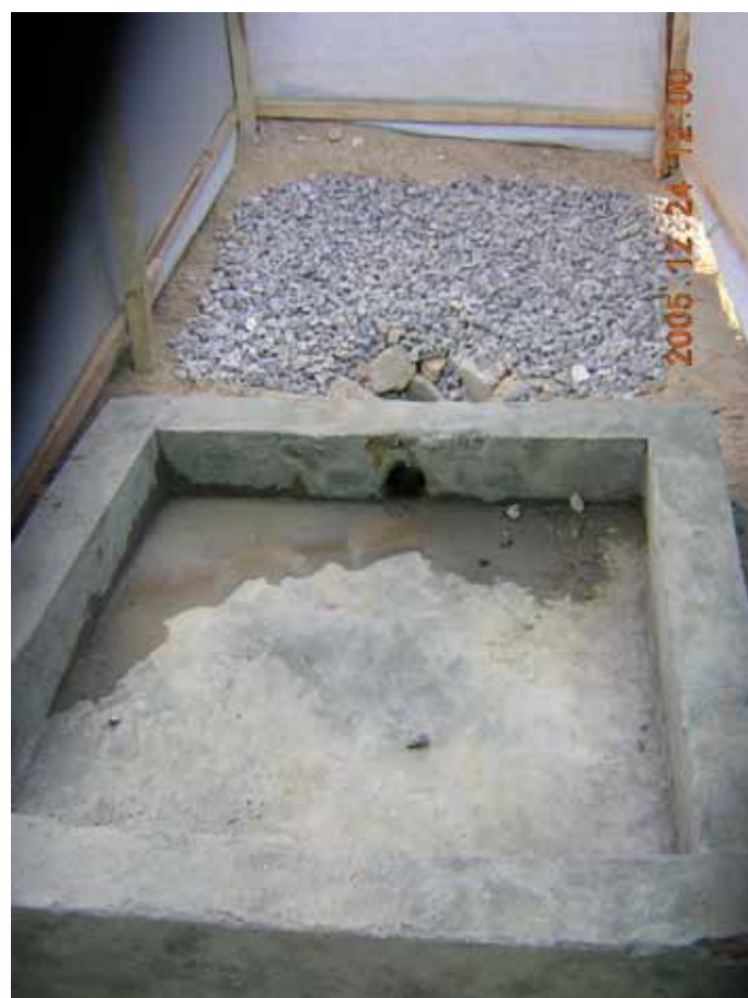
Private washing slab for washing sanitary cloths
