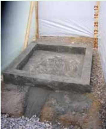
Sanitary pad washing slab inside screened unit
