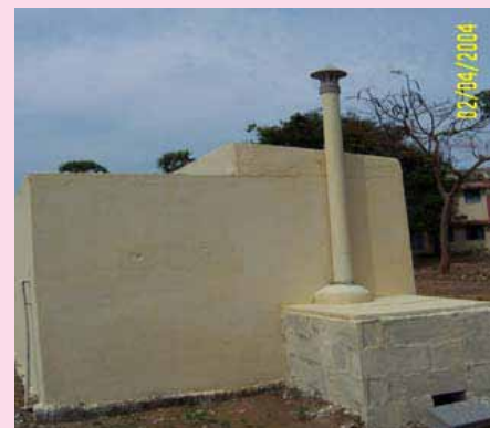
External view of the latrine and incinerator
