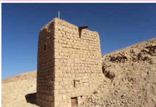
Raised urine diversion pit latrine with urine pipe exit exposed to the atmosphere, Afghanistan (Photo: ACF, Afghanistan)
