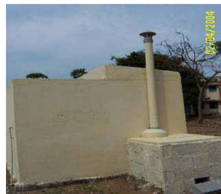
External view of the latrine and incinerator
