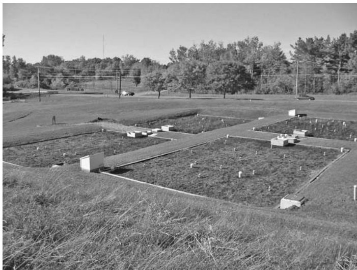
FIGURE 7.2 Four-cell HSSF wetland at the University of Vermont. White pipes extending from the wetland beds are sampling ports.
