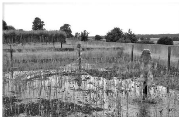
FIGURE 1.20 Biosolids mineralization reedbeds at Skovby, Denmark. The bed in the foreground is newly excavated and replanted, and is receiving initial doses of biosolids. The bed in the left background is a mature stand of Phragmites that has been receiving biosolids for several years.
