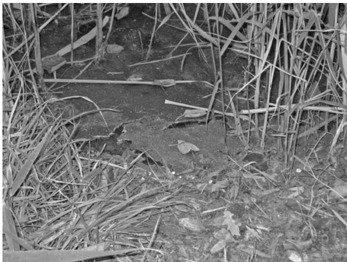
FIGURE 7.31 Accumulated particulate organic matter on top of an intermittent downflow VF wetland bed in Roussillon, France.
