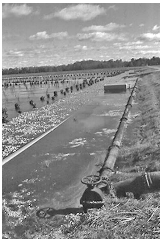
FIGURE 2.28 The flooded inlet zone of the Denham Springs, Louisiana, HSSF wetland.
