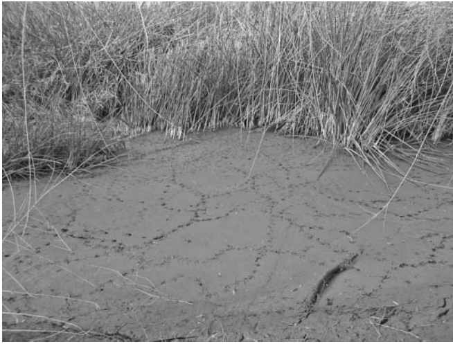
FIGURE 7.13 Excessive TSS can fill the inlet deep zone to a treatment wetland, as happened at the Tucson, Arizona, sweetwater wetland. Note the bird tracks that highlight the complete filling of the deep zone with relatively high density solids. Incoming waters had high TSS from filter backwashes at the secondary treatment plant that provided the source water.
