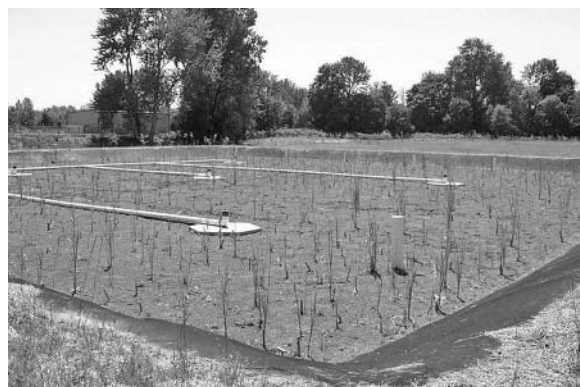
FIGURE 1.14 The Salem, Oregon, VF system just after planting. (Photo courtesy of the city of Salem.)
