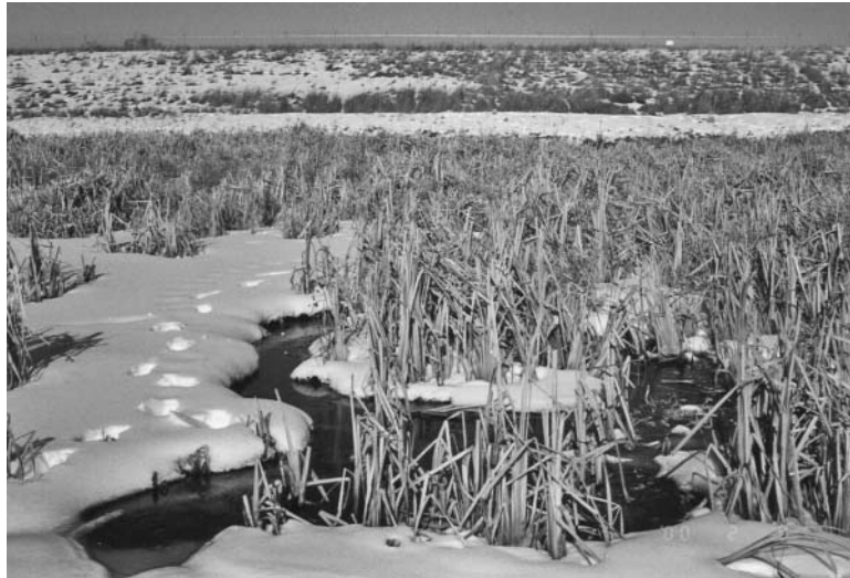
FIGURE 4.26 Winter conditions at a constructed FWS wetland near Hillsdale, Michigan. Note the snow that is held up out of the water by standing dead and litter.
