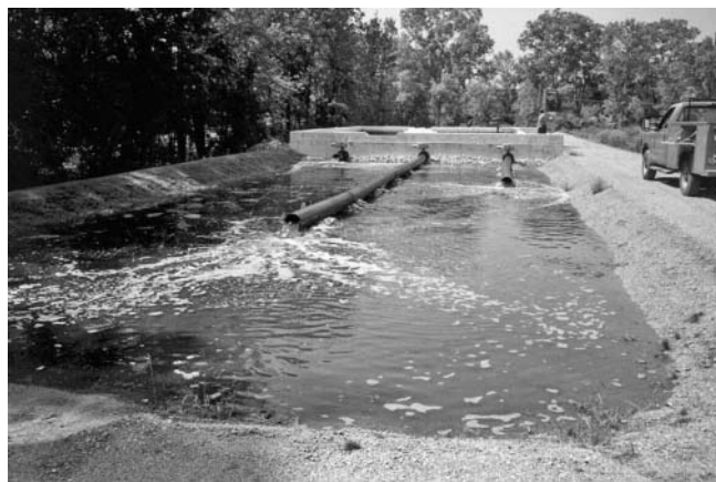
FIGURE 2.33 The flooding of the vertical intermittent sand filters at the Saginaw, Michigan, landfill leachate treatment system. Water is dosed twice per day, with each flooding lasting only a few minutes. Rip-rap splash pads prevent erosion for the three-point distribution.
