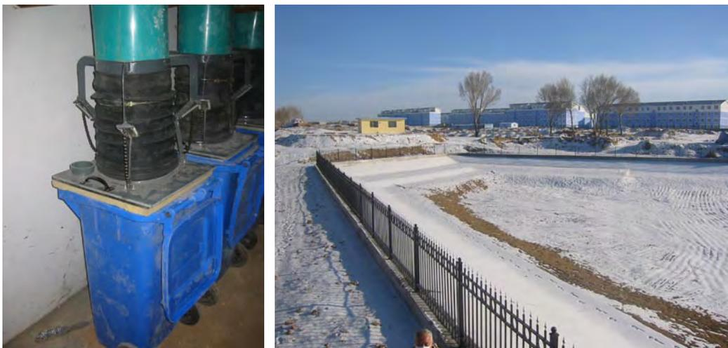
(left) Bins in basement containing dry faeces mixed with dry cellulose fibre – drying & bulking agent & carbon source for later composting
