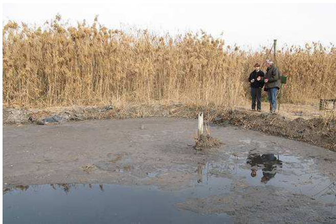
Fig. 10: Foreground: primary sludge drying bed (was: reed bed for primary sludge conversion to soil). Background: reed beds (source: E. v. Münch, Jan. 2009)
