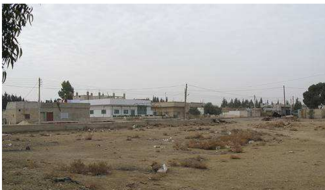
Fig. 4: View of village Haran Al-Awamid (viewed from wastewater treatment plant). Source: E. v. Münch, Jan. 2009.
