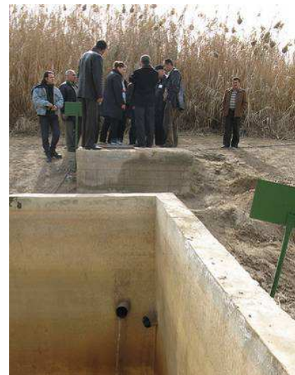
Fig. 12: Foreground: effluent tank with two effluent pipes discharging from the two reed beds. Background: reed beds and group of trainees (source: E v. Münch, Jan. 2009).
