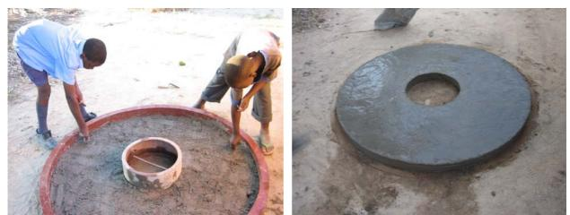
The 3mm steel reinforcing wires are added in a grid formation. Then the second half of the concrete mix added and smoothed off. The shuttering is then removed. This is allowed to harden overnight and then kept wet under a plastic sheet or wet sand for a week before moving.
