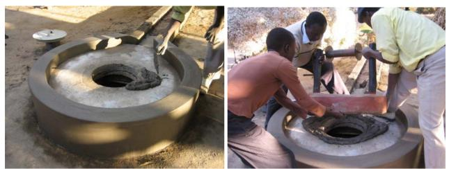
Once the raised collar system was been removed and the well cover cleaned down some strong cement mortar is laid down around the well access hole for the windlass system to lay in.
