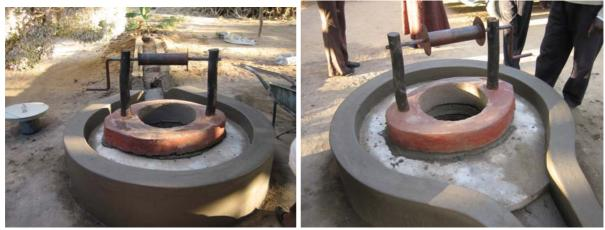
The windlass system is mounted around the well access hole leaving enough room on either side to allow water to drain away down into the run off system. A further layer of mortar is added to the well slab and finishing touches are made all over the well to make it neat, strong and tidy. The new upgraded family well can then be put to use.
