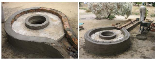
The well head and run-off are plastered with strong cement mortar
