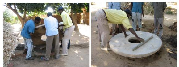
The new well slab is placed over the original well slab in a bed of cement mortar. The slab level is adjusted so it slopes very slightly towards the side where the runoff will be built.
