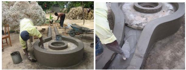
The strong mortar work extends down the slope leading from the slab to the water run-off channel.
