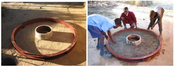
The shuttering is laid down on level ground overlaid by sand which is wetted. Half the concrete mix is added and levelled off.
