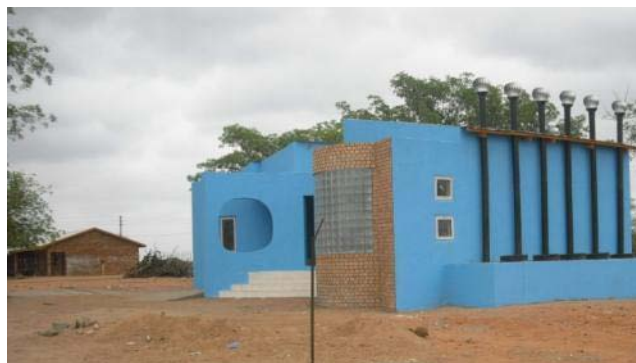
Figure 4: The Baranuka High School (in Lulekani, South Africa) toilet block that was built by The Clean Shop and Trevor Mulaudzi and serviced by the school (source: T. Mulaudzi, 2008)
