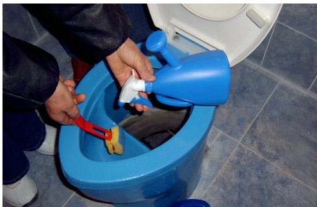
Figure 7: Cleaning a UDDT in a public cultural house in Stara Zagora, Bulgaria. Project was implemented by Earth Forever Foundation and WECF (source: WECF, M. Torres, 2008).
