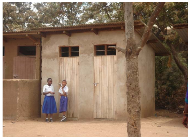
Figure 2: School toilet in Tanzania: The special needs of girls and women during the time of menstruation – such as privacy, facilities for disposal of sanitary materials – must be brought to the forefront (source: M. Sommer, 2009).
