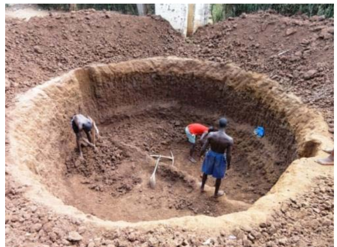
Figure 1: Excavations for a biogas digester in Livingstone, Zambia at a project of the Devolution Trust Fund (DTF) (source: P. Feiereisen, 2011)
