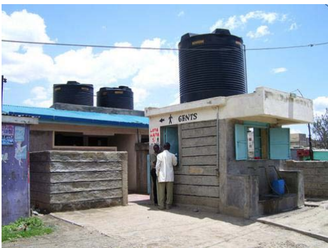
Figure 6: Naivasha public toilet with water kiosk. In front is the water kiosk that functions as an operator room. Customers pay at the side window, where the two people are standing. Behind them the gents section of the toilet can be seen (source: C. Rieck, 2008) 3 .
