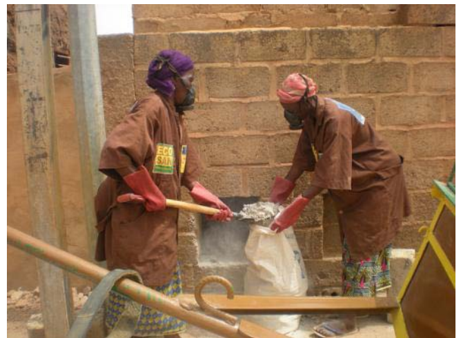
Figure 1: Two staff members from a service provider are emptying the faeces vaults of household UDDTs in Ouagadougou, Burkina Faso (source: S. Tapsoba, 2009) 1 .
