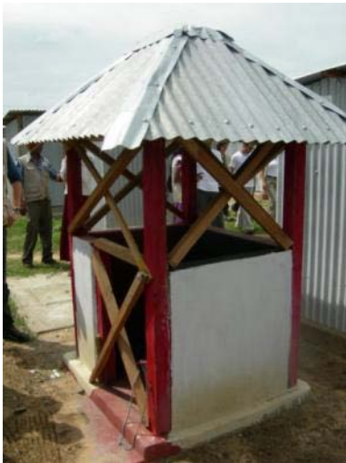
Figure 4: Child friendly toilet which is open and bright for use by young children in a post Tsunami camp in Sri Lanka in 2004 (source: J. Lapegue, ACF, 2004).
