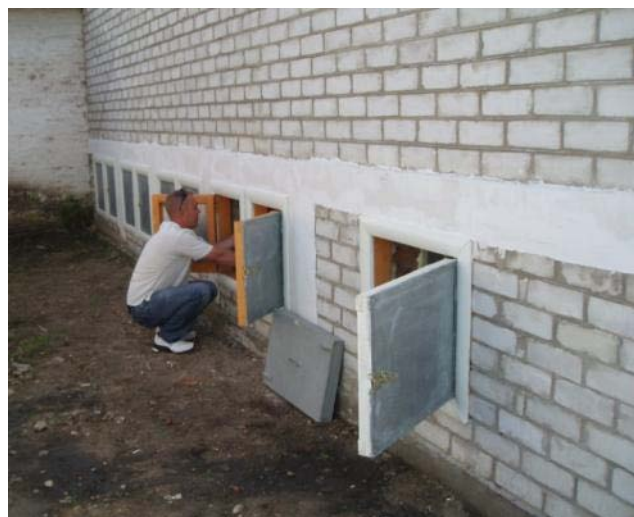
Figure 8: Inspection of the faecal chambers of a UDDT school toilet block in Nizhyn, Ukraine, constructed by the local NGO Mama86 (source: WECF, C. Wendland, 2010).
