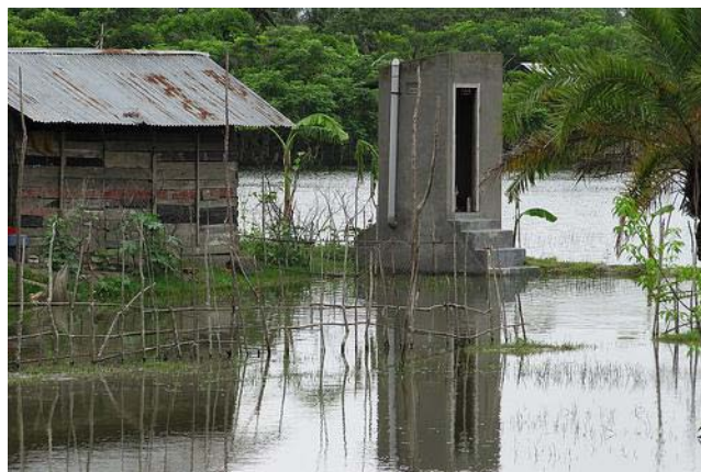
Figure 1: Urine Diversion Dehydration Toilets (UDDT) withstood the flood waters that resulted from a cyclone that struck southern Bangladesh in 2009 (source: A. Delepiere). More photos from this project: www.flickr.com/photos/gtzecosan/sets/72157626407064863/
