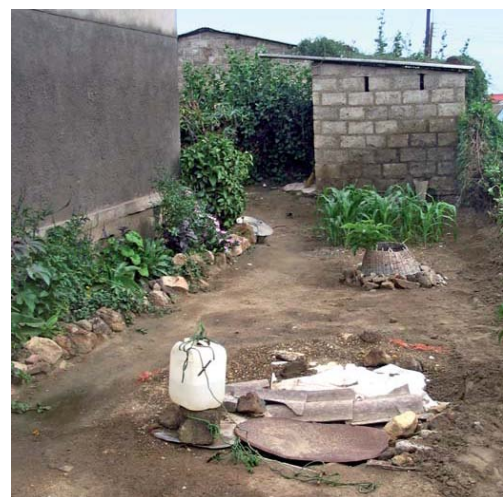
Figure 1: Unprotected well at close distance of a pit latrine in Lusaka, Zambia (source: K. Mayumbelo, 2006).
