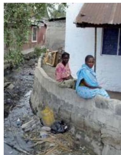
Figure 5: In densely populated areas infiltration of wastewater threatens groundwater resources in Senegal. Note also the water pipe in the drain which is a common but unsafe practice (source: BGR, 2005).
