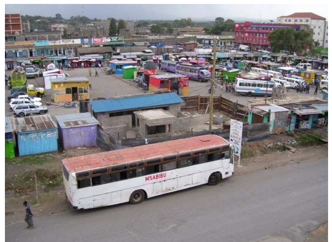
Fig. 3: View of Naivasha bus park with the public toilet at the front of the plot (behind the large bus); during the construction in mid 2007. All photos in this document by C. Rieck (GTZ) in 2008/2009.
