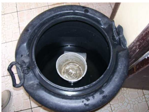
Fig. 7: Pour flush system with small bucket (2-4 L) in drum. The small bucket is used to flush the toilet.
