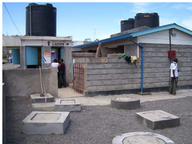
Fig. 3: New public sanitation facility with water kiosk (left side). Underground biogas plant in front.
