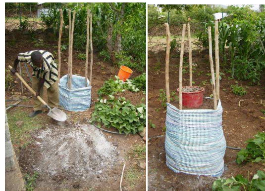
Fig. 5: 1 (left) Mixing soil, compost and ash to fill the tower and 2 (right) Filled greywater tower.
