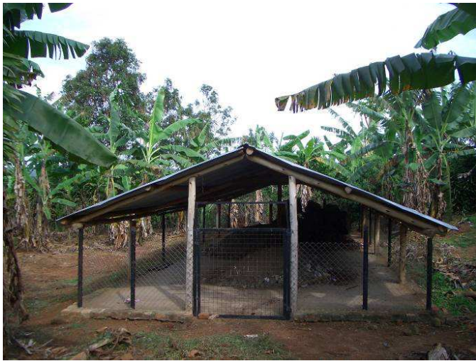
Figure 2: Treatment area for faecal matter, Kalungu School, Uganda.
