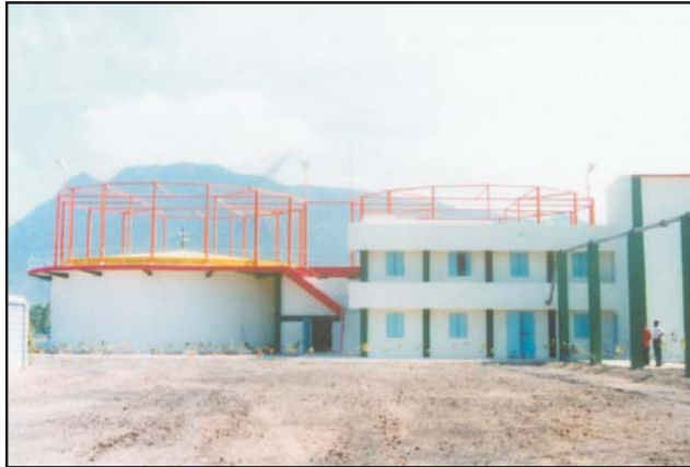
View of the Biomethanation Plant
