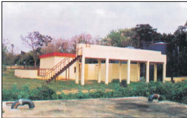
Sump & Pump House, Control Room and Grit Chamber
