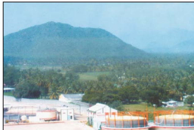
Overall view of the plant
