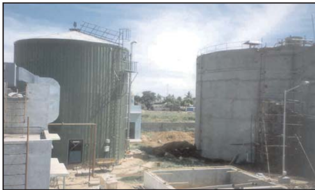
Overall view of the Plant
