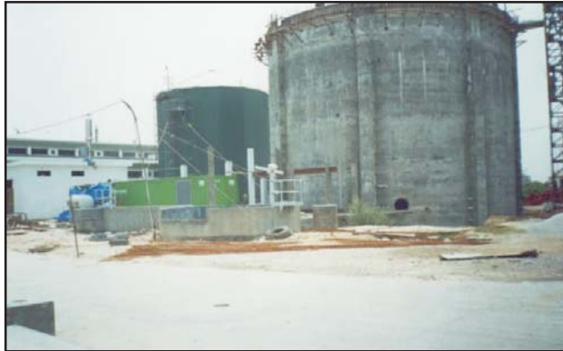
LSATR Digester and the Gas Holder
