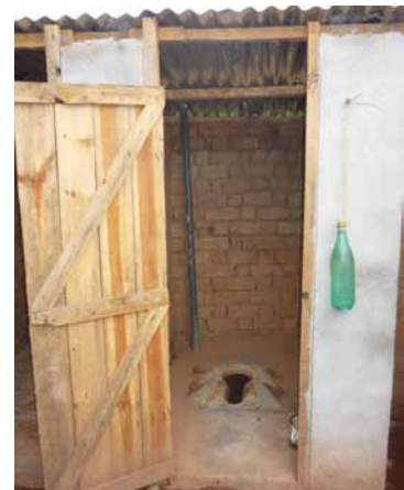
GSF programmes help raise awareness about sanitation and hygiene and create demand for toilets.
