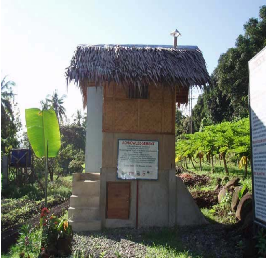
Ecosan double vault urine-diversion dehydration toilet (UDDT) at PUVeP, Manresa Farm, Cagayan de Oro City
