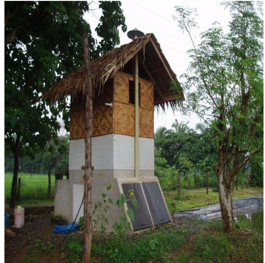
Ecosan double vault urine-diversion dehydration toilet (UDDT) at PUVeP, Manresa Farm, Cagayan de Oro City
