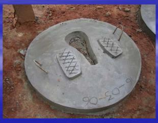
3. The double pit composting toilet known as the Fossa alterna alternates the use of two shallow pits where compost is produced and dug out.
