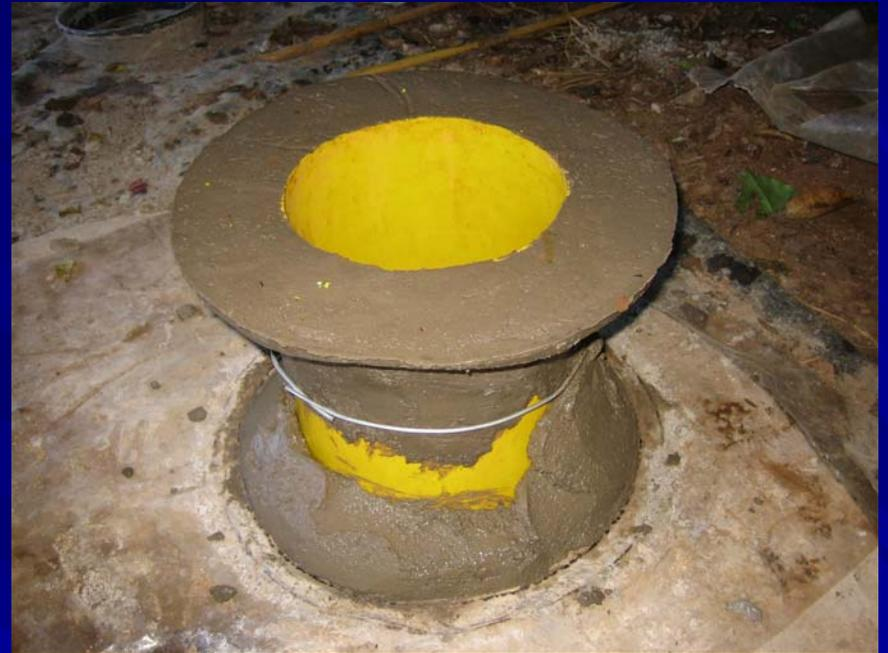
**This ring of concrete will become the seat of the pedestal. Additional concrete is then added half way up the side wall of the bucket. This is covered with a plastic sheet and allowed to cure for 2 days. The following morning the concrete is wetted down and a ring of 3mm wire prepared and wound around the middle of the bucket. The bucket is then carefully turned over.**
