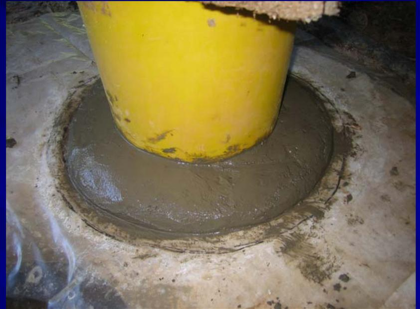
**A mix of cement and river sand is now made up. If Portland cement is used the mix is 1 part cement and 3 parts river sand. If masonry cement is used a 1:1 mix is used. The concrete can be mixed in small lots with a litre of cement being mixed with the sand at any one time. The concrete is made into a neat round shape with a trowel. A ring of 3mm wire is placed inside the concrete.**
