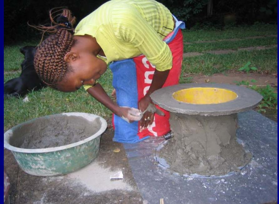
**After a full day of curing the bucket is turned over and placed back on the plastic sheet. More concrete is missed and built up around the base and also around the side walls of the bucket and around the plastic pipe. The concrete is then allowed to set overnight and then is cured over the course of a week or more. It is kept wet at all times to allow the concrete to develop full strength.**
