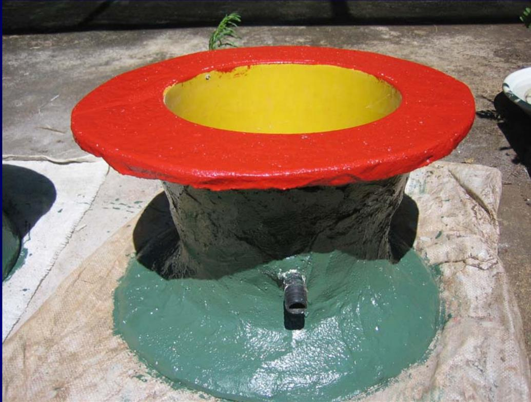
**After this the concrete can be painted with brightly coloured enamel paint. The unit will still work if not painted, but is more attractive if brightly coloured. The urine pipe placed above slab level makes it possible to divert the urine to a tree or plastic container even when the toilet is placed over a pit.**
