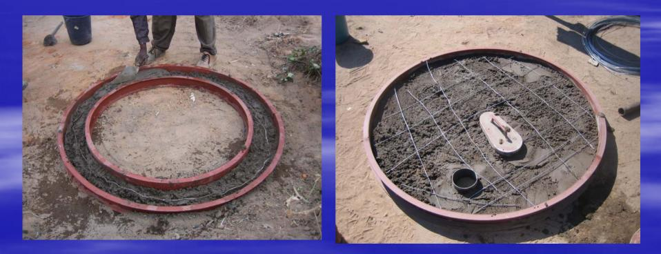
The three concrete pieces are left to harden and cure for several days. The soil within one ring beam which will be used for the toilet is now dug down to 1.5m with the second dug down to 0.3m.
