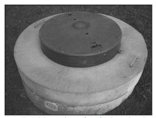
Above: New style vermin proof cap for dug or bored wells. Below: Vermin proof cap for drilled wells.
