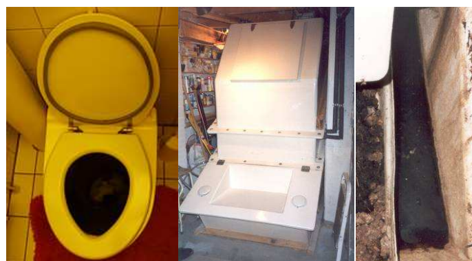
Fig. 6: Berger Terra Nova composting toilet system with toilet pedestal (left) and composting container (middle). Separation chamber inside the bottom compartment for leachate (right). Source: A. Schöpe, 2009 (left) and Berger Biotechnik.
