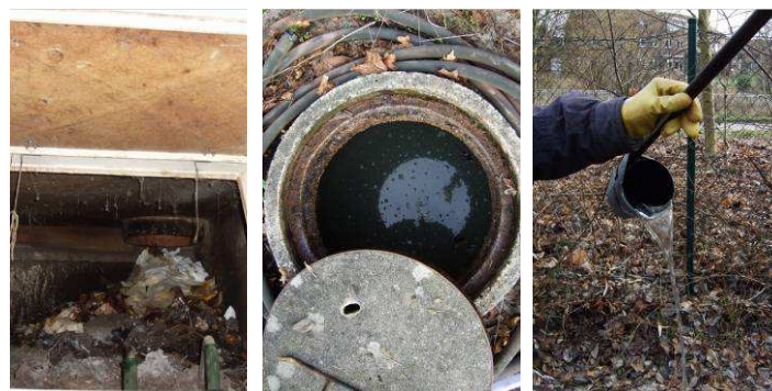
Fig. 10: Compost heap inside the composting container of the toilet (left), greywater in Imhoff tank (middle) and final effluent from constructed wetland (right). Source: A. Schöpe, 2009.
