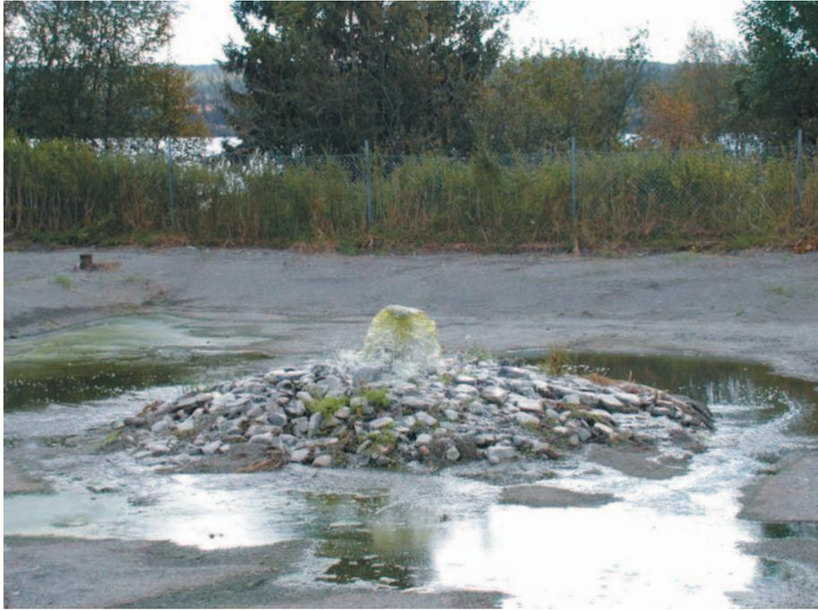
Figure 12. Open sand filter bed in Alsen, Krokoms municipality in Sweden. Pre-treated wastewater is distributed on the surface by flooding (Photo: E. af Petersens).
