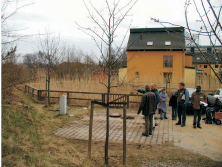
Figure 9. Vertical soil filter planted with common reed used for greywater treatment in an ecological residential area, Hamburg, Germany. The water is applied from the top and percolates vertically through the bed in an unsaturated flow. The dimensioned load is 60 l/m<sup>2</sup>/day (photo: P. Ridderstolpe).
