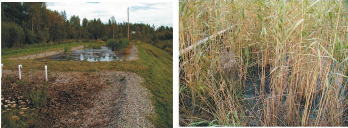
Figure 17. Sludge drainage beds are a well-proved method for sewage sludge management. With the planting of plants (e.g. common reed) a valuable humus soil is produced.
