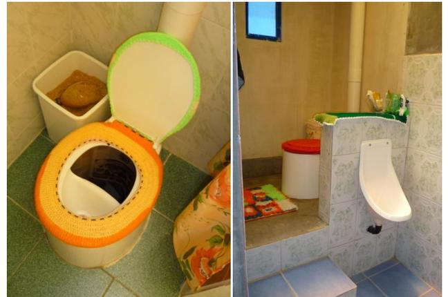
**Fig. 9:** View of the interior of the UDDT unit. Right picture shows also the urinal (Andersson, 2011).
