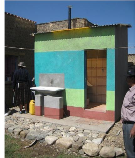
**Fig. 8:** Front view of the UDDT unit with handwash basin on the outside (Andersson, 2011).
