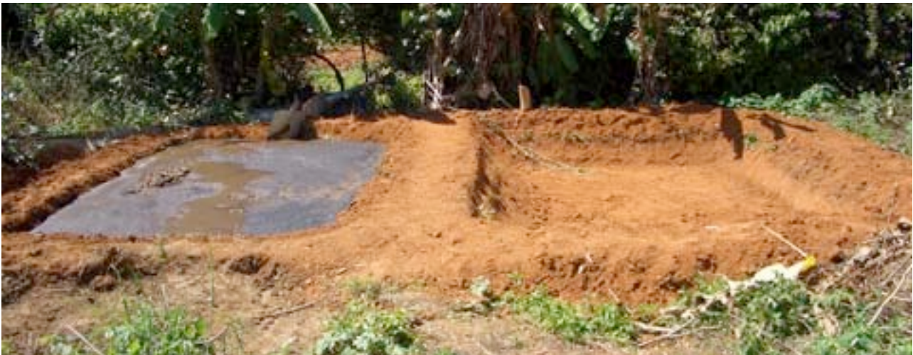
figure 13: View of simple sludge drying beds
