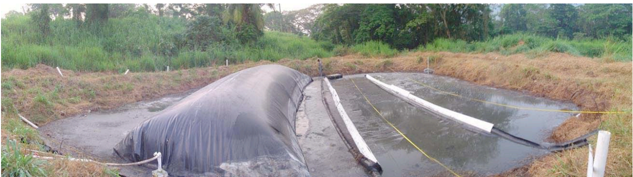
figure 7: Anaerobic lagoon with recovery of biogas
